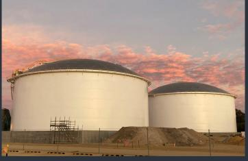
A 3-coat Sherwin Williams (now Hempel) system consisting of an Organic Zinc Rich primer, Epoxy build coat & an Acrylic Urethane top coat was applied to the tank externals shell.
