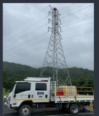
The transmission line is approximately 5.5km in length, consisting of 14 tension and 4 suspension structures constructed between the Kamerunga Substation and the Barron Gorge Hydro-electric Powerstation in the Cairns region, Far North Queensland.
